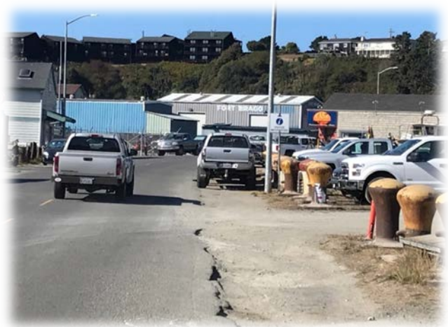
Shoulder of North Harbor Drive
