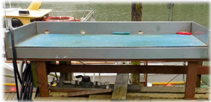
Existing North Side Fish Cleaning Station
